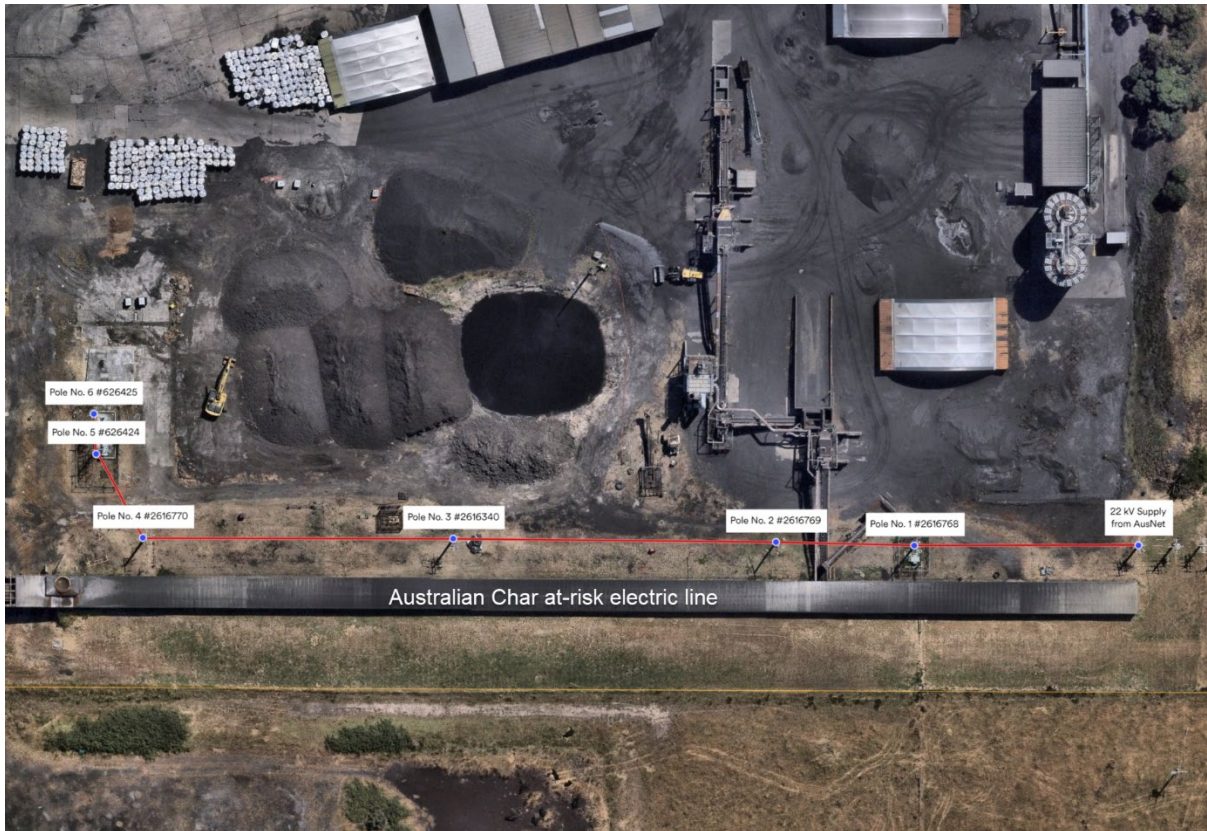
(Figure 2 – Image detailing Australian Chars’ at-risk electric line)
